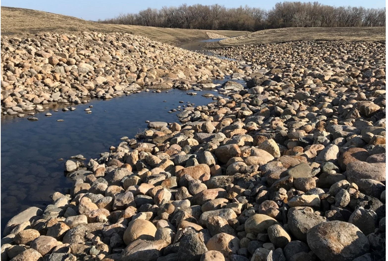
Close up view of a rock riffle in Phase 1. Photograph courtesy of Robert Sip, RRWMB Executive Director – April 22, 2021.
