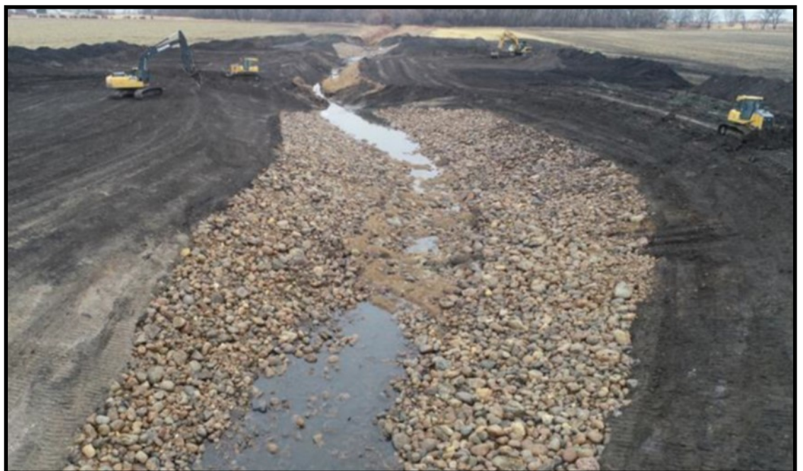
Phase 1 construction in November 2020. Photograph courtesy of the BdSWD.
